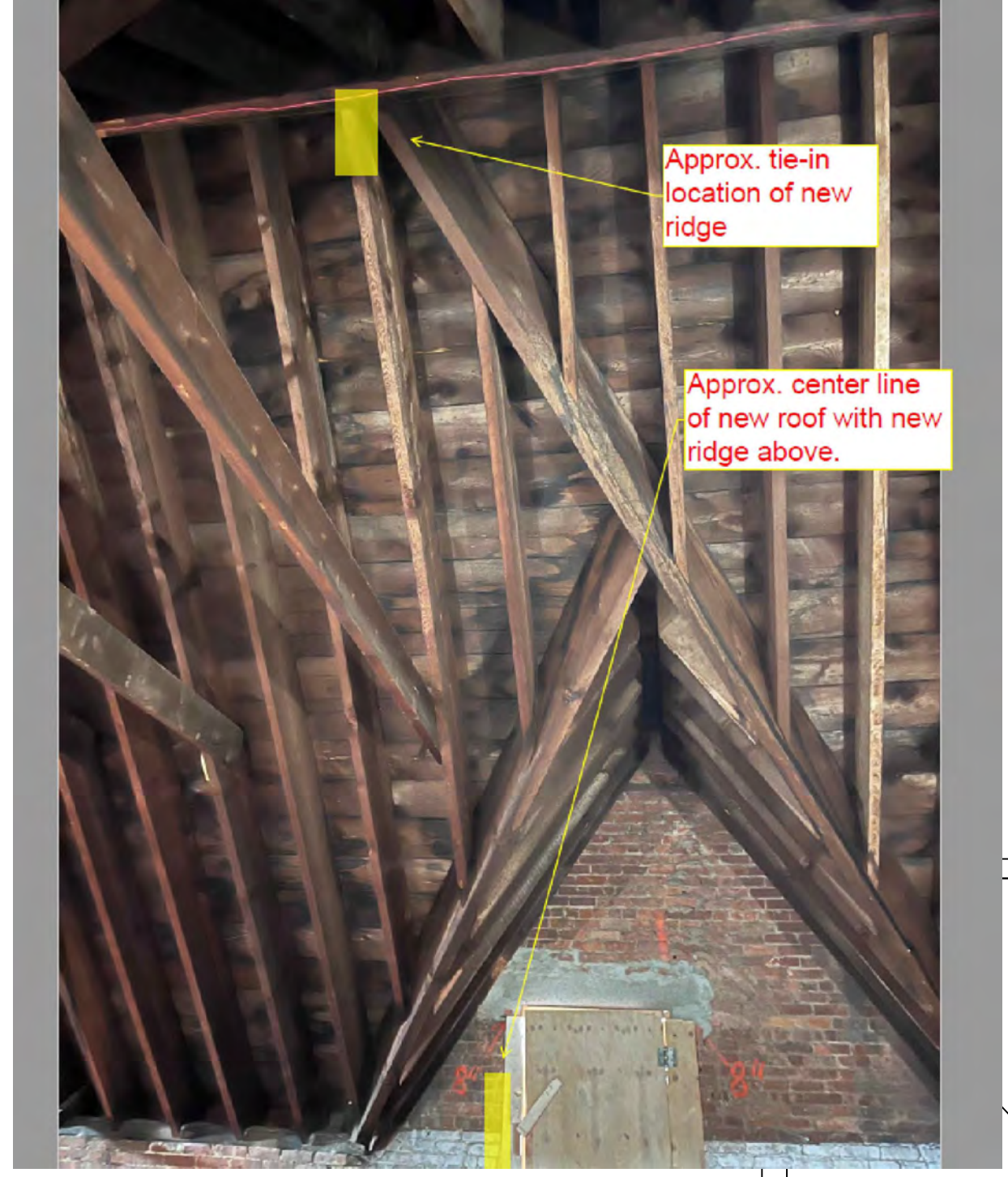
EXISTING PHOTO - 2 UNDERSIDE OF THE ROOF SHOWING JOIST
