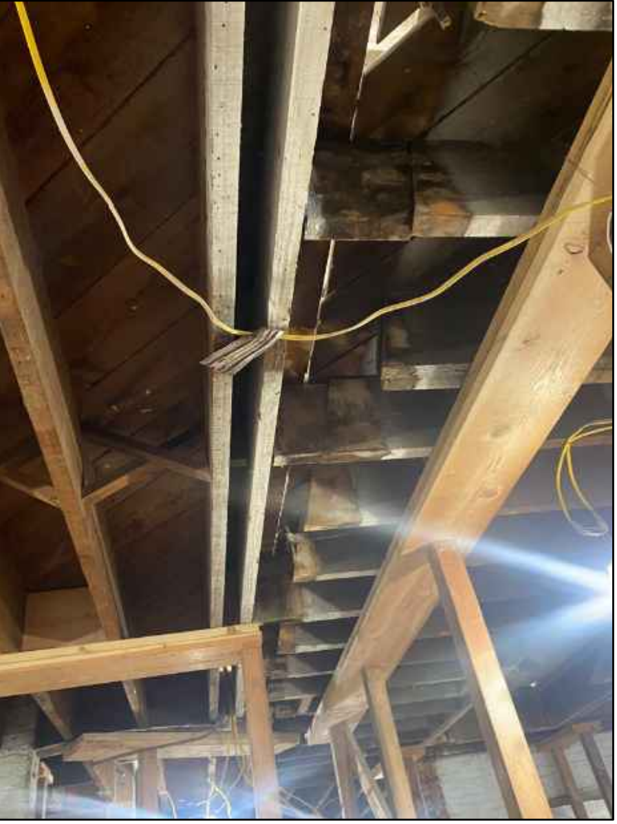
EXISTING PHOTO-1 DECK SUPPORTING ANGLES REQUIRED L 6X6 1/2 CONT. 3/4" HILTY HIT HY 70 ADHESIVE ANCHOR @ 2'-0" WITH 6" MIN. EMBEDMENT (PERIMETER OF ELEVATOR LOBBY)
