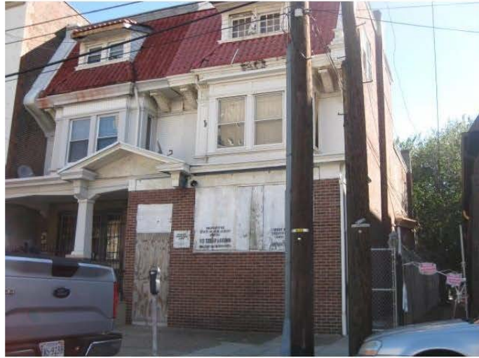
Front view of the subject (from N. 7 th Street)
