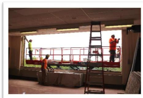
*Workers reconstructing window frames to allow for the installation of new windows.*
