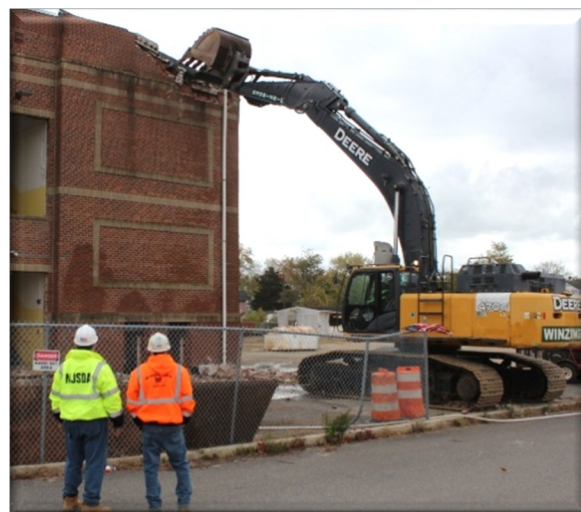
Construction team observes demolition activities during the early site preparation/demolition event for the new Decatur Avenue School in Pleasantville.
