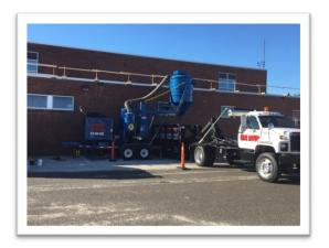
Construction activity began on the Bridgeton Senior High School emergent project during the reporting period. This \$9.8 million project will consist primarily of a roof replacement to remedy water infiltration concerns. It includes replacement of 160,000 square feet of roof and minor masonry repairs. This work is anticipated for completion by the start of the 2021 school-year.
