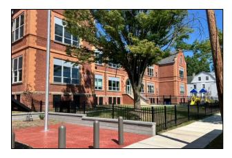
The SDA's addition/renovation project at the Cleveland Street Elementary School in Orange included an 11,500 square-foot addition and renovations to the 100+ year-old existing facility. The renovations included converting the basement areas to provide a main office, a media center, an art room, a music room, a science room, and a computer instructional area. It also included replacement of windows throughout the
