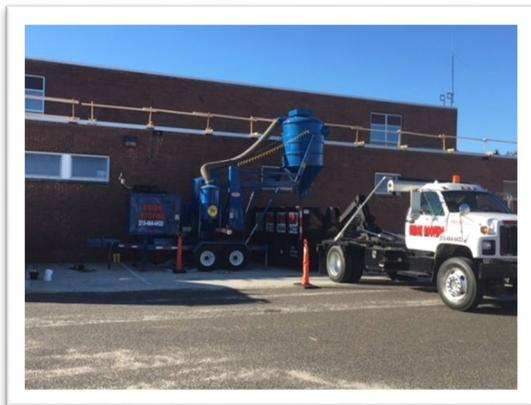
Construction activity began on the Bridgeton Senior High School emergent project during the reporting period. This \$9.8 million project will consist primarily of a roof replacement to remedy water infiltration concerns. It includes replacement of 160,000 square feet of roof and minor masonry repairs. This work is anticipated for completion by the start of the 2021 school-year.
