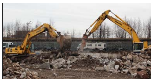
Demolition activities at ES 3
